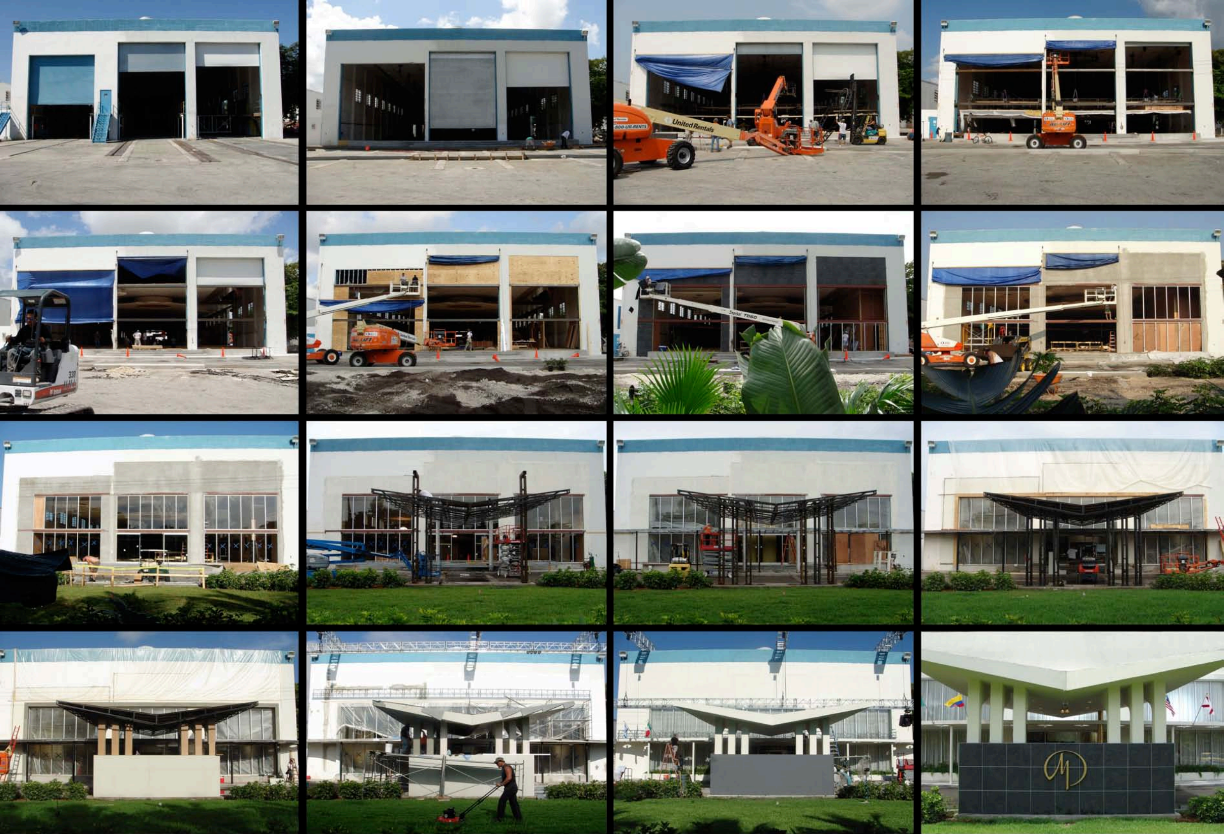
An existing warehouse with three bays of steel roll-up doors and a parking lot was transformed into the glamorous Miramar lobby entrance with a porte cochere, covered walkways, new driveway and a landscaped roundabout.
